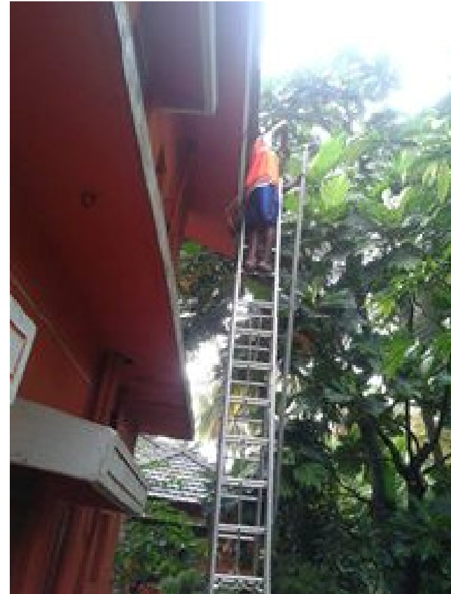
Worker fixing the mosquito trap on top of the pipe
